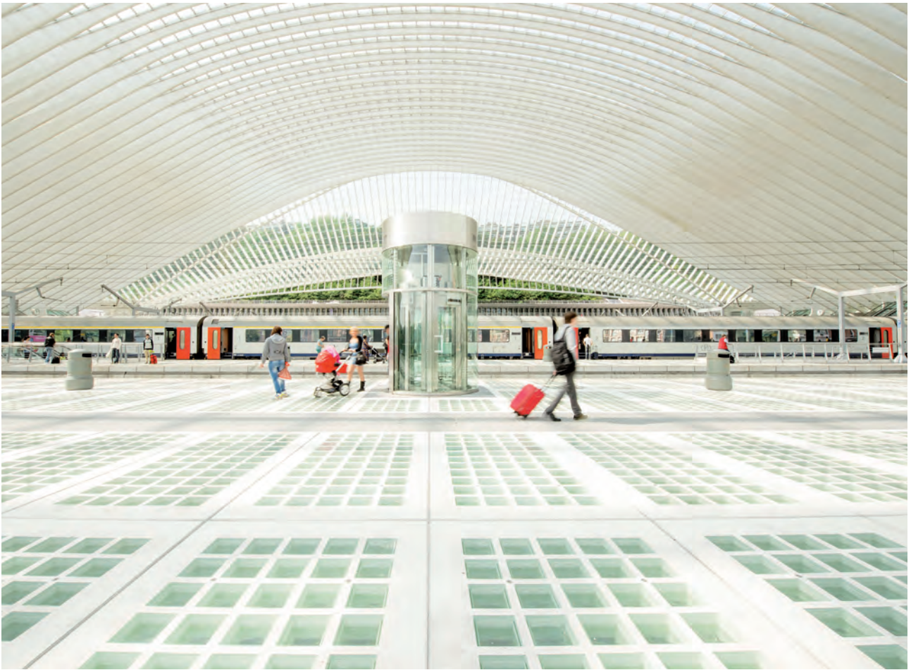
In Liège, one of the world's most beautiful train stations, truly sculpted into the urban space by Santiago Calatrava.
